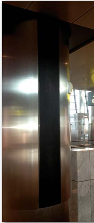
Renkus-Heinz Iconyx speakers installed at Doha's new terminal
