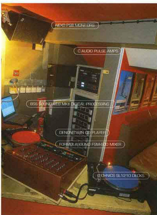
The backroom equipment at Plastic People includes C Audio Pulse amplification and BSS's new Soundweb MkII digital signal processing, used to control Funktion One speakers as well as dedicated controllers for the Nexo PS10s used for peripheral sound
